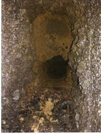
Figure 22 Trench BP 44 (Part 2)
